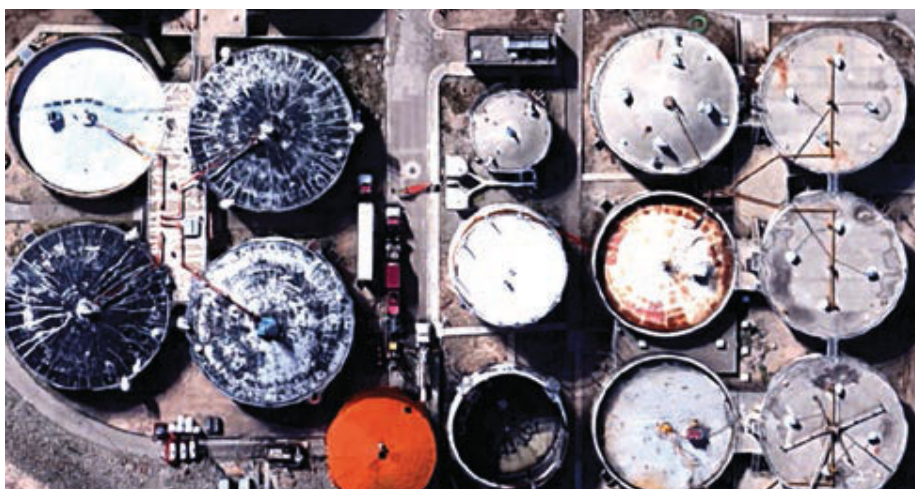
A water resource recovery facility in New Mexico meets 95 percent of its energy demand using onsite solar power and biogas generation. Photo by Drylet LLC
