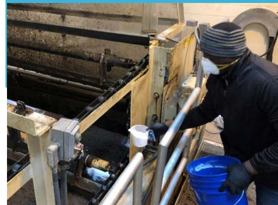
Product dosing into the thickened sludge feed to the primary digesters.
